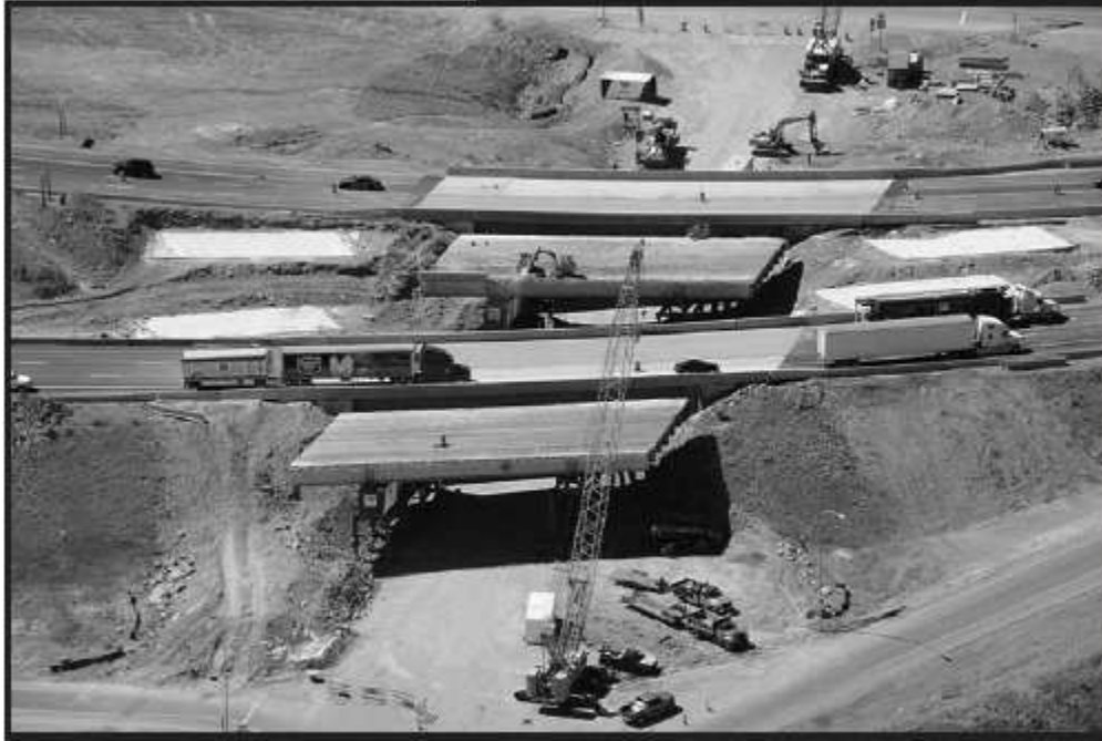
Figure 1.6. Lambs Canyon Bridge constructed using ABC methods (FHWA, 2010)
