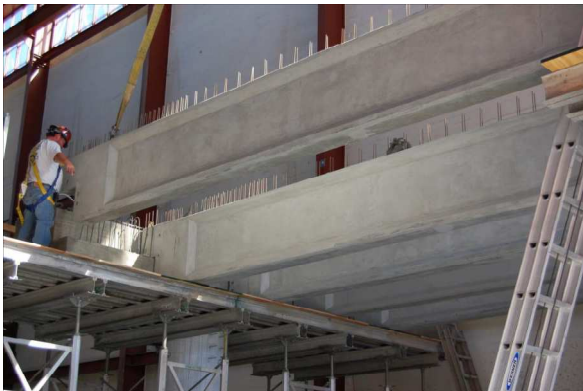
(a) Installing as-built girders
