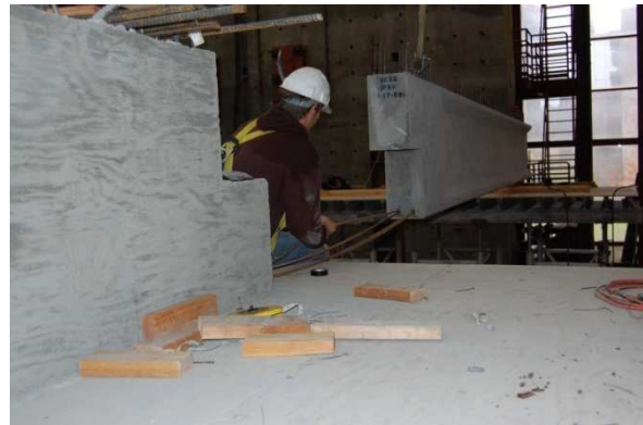
(b) Installing strand for improved girders
