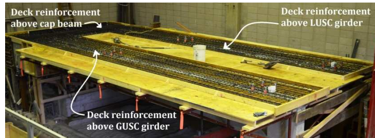
c. Deck formwork and reinforcement
