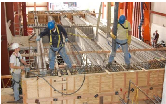
(c) Casting an abutment
